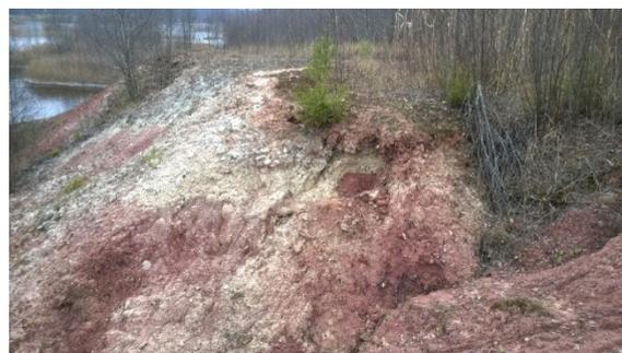
Fig. 3. Dolomite landslips in the Kuprava quarry wall.
