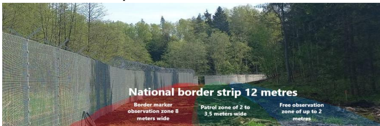
Fig.1 State border strip of the Republic of Latvia, 12 meters wide, with zone divisions (created by the authors)
