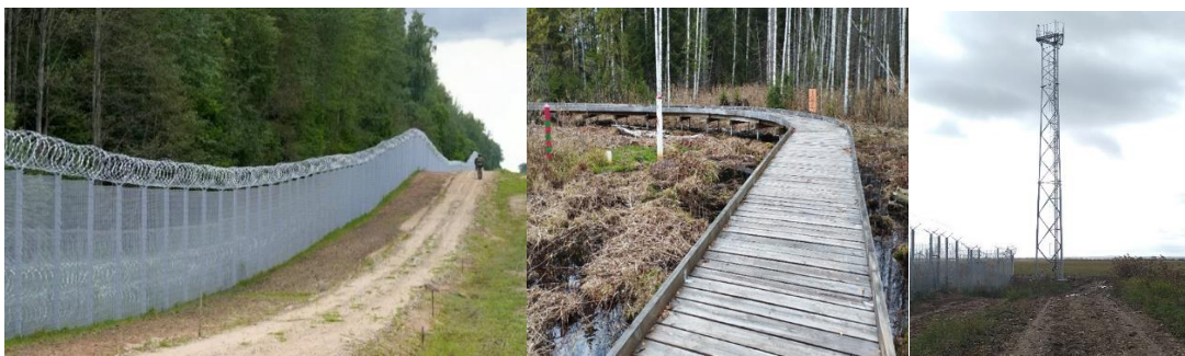
Fig.1 Fence and infrastructure elements (border guard unpublished image, 2023)
