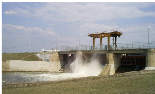
Fig. 3. Water flow through the supercharger dam of Nugushskiy water power development [13]
