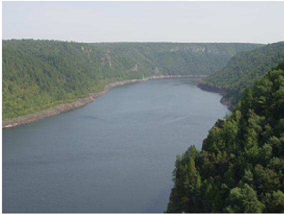
Fig. 6. A view of Umaguzinskiy water reservoir (photo taken by the author)
