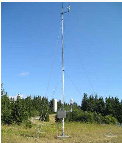
Figure 3: Mast of LMS Rozhen - Gamma probe and Meteo station
