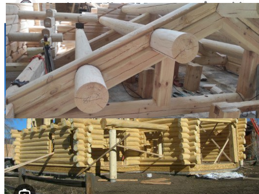
Fig. 9. The structural elements of the log house
